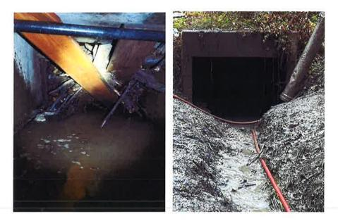
The pictures show an example of why developing an ordinance and educating the public about stormwater drains is important. This is a stormwater culvert that Ace recently cleaned out and it was filled with debris. When storm drains become blocked like this, it can lead to flooding and standing water. These kind of materials should not be in a storm drain.
